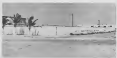
New fence wall section from Gate 1 to Coruba Supermarket. Muraya nobo for di Porta No. 1 te na Coruba Supermarket.
